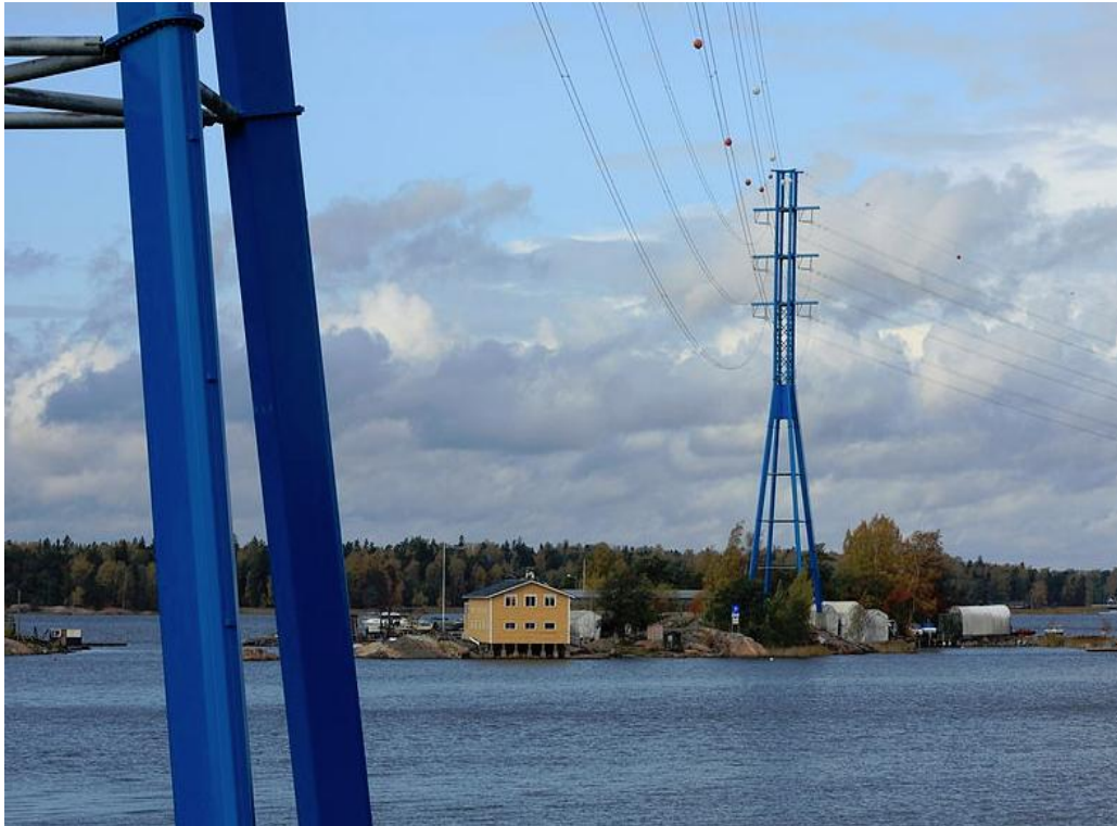
Figure 7: Salmisaari-Meilahti transmission lines in Helsinki. These are 60-meter landscape towers, designed by Antti Nurmesniemi. 23
