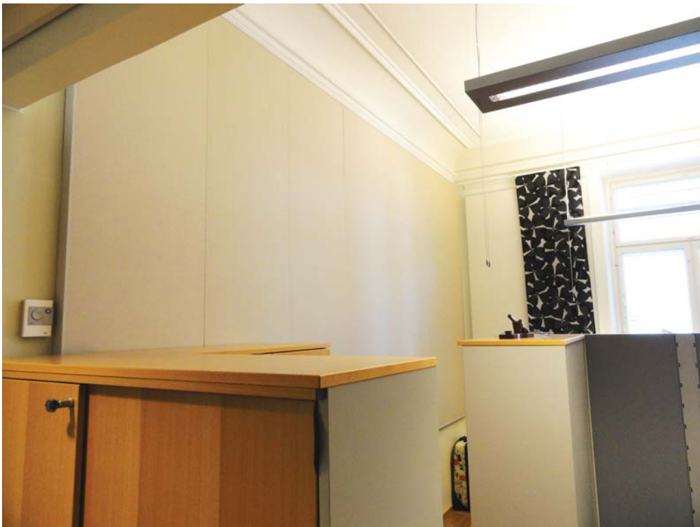
(b) Absorptive wall panel installed to two-person office room 339.
