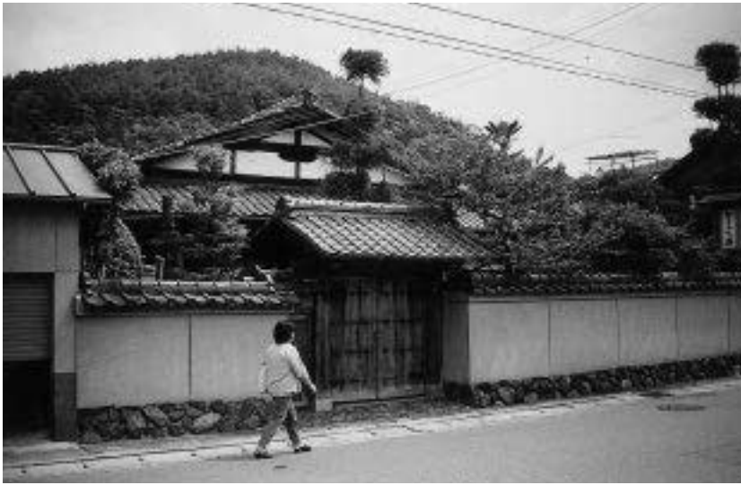
FIG.35 KAMIGAMO SHAKEMACHI. ONE OF KYOTO'S HISTORIC PRESERVATION AREAS WITH RESIDENCES FOR SHINTO PRIESTS. RS.
