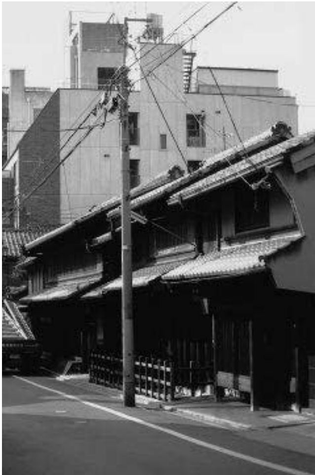
FIG.52 VIEW FROM YATACHŌ. IN THE FOREGROUND THE SUGIMOTO HOUSE. RS.
