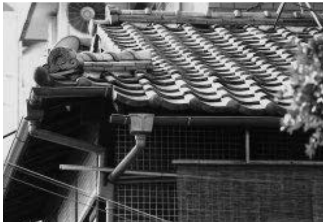
FIG. 63 TILE ROOF, SHINKAMANZACHŌ. RS.
