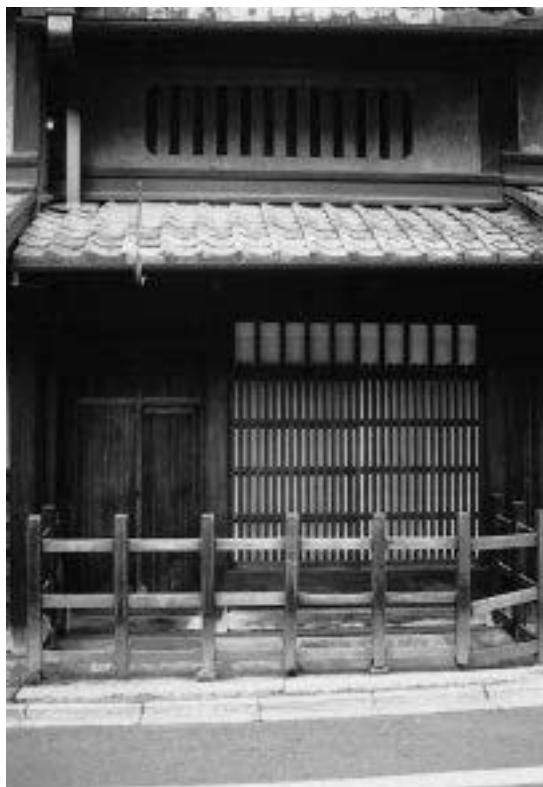
FIG.58 TSUSHI-NIKAI MACHIYA. THE TRADITIONAL KYOTO TOWNHOUSE WITH 1.5 FLOORS AND WITH A WELL-PRESERVED LONG MUSHIKO MADO, INSECT WINDOW, IN THE UPPER FLOOR. YATACHŌ. RS.
