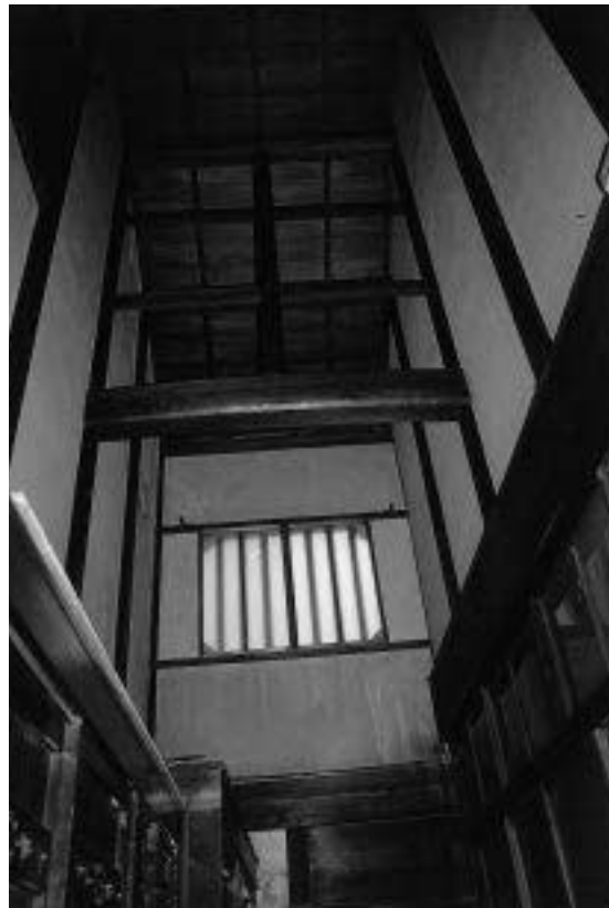
FIG.77 INTERIOR OF THE NAKA HOUSE. VIEW OF THE EARTH FLOOR CORRIDOR, TŌRINIWA. THE STRUCTURAL PARTS SHOW A SOPHISTICATED WOODWORK WITH A COMBINATION OF DIFFERENT WOODEN MATERIALS. RS.
