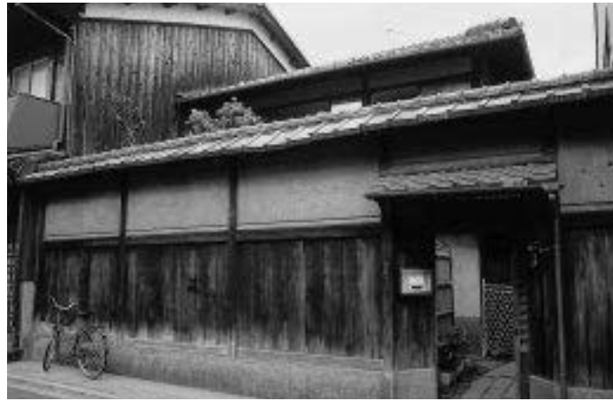
FIG.75 FACADE OF THE KOBAYASHI HOUSE. SHIMOTAYA STYLE, THE HOUSE IS RECESSED FROM THE STREET. NOTE THE HIGH WOODEN FENCE, TAKABEI, AS A HALLMARK OF THE STYLE. RS.
