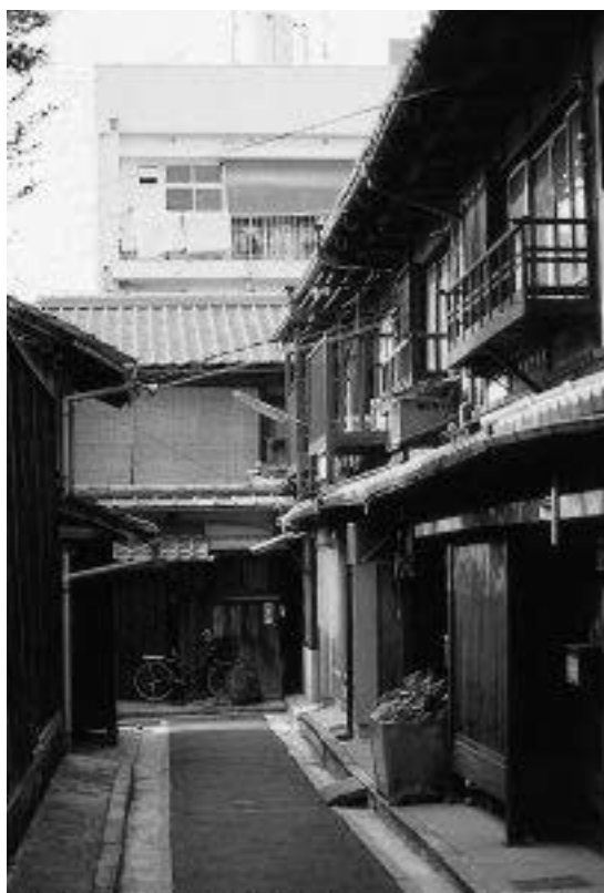
FIG.30 SHINKAMANZACHŌ. A NARROW URBAN LANE THAT IS ILLEGAL ACCORDING TO THE FIRE PREVENTION STANDARDS. ONE OF THE THREE NEIGHBOURHOODS THAT WAS MEASURED BY THE AUTHOR FOR THE SURVEY. RS.
