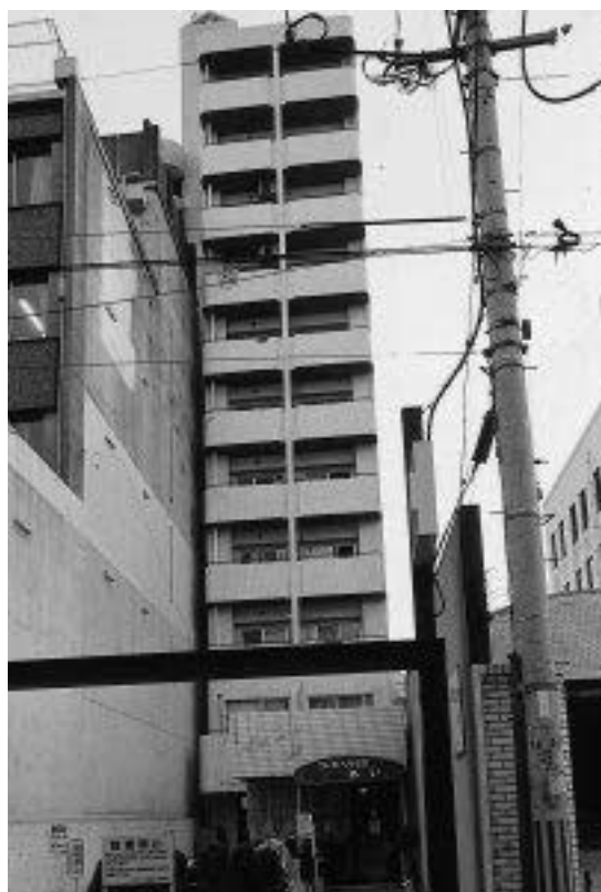
FIG.31 URBAN TRANSFORMATION PROCESS PROGRESSING IN THE CENTRAL AREA. BECAUSE OF THE LIGHT ANGLE REGULATIONS, THE HIGH-RISE BUILDING MUST BE RECESSED FROM THE STREET LINE. RS.
