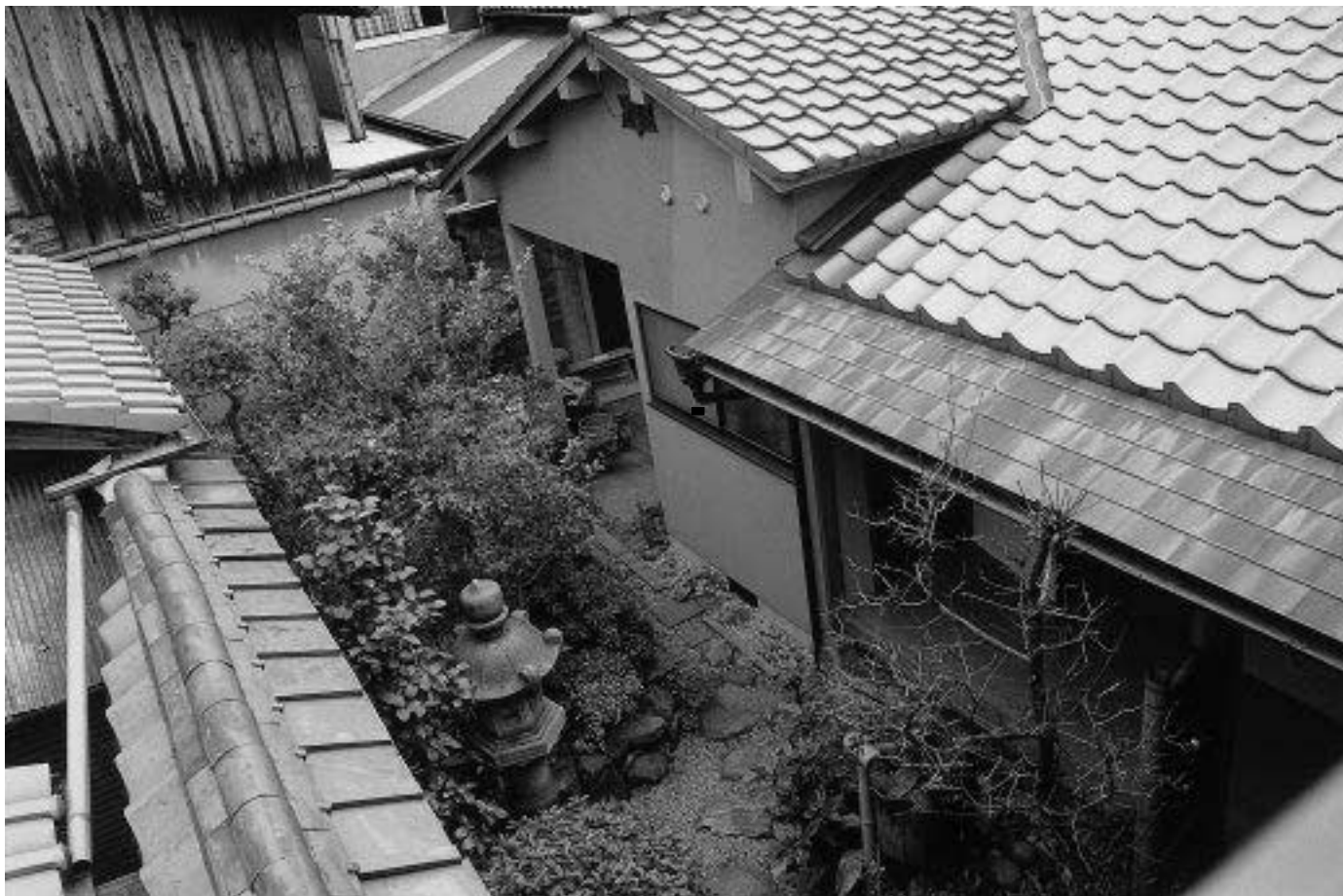
FIG.79 GARDEN OF THE MATSUMOTO HOUSE WITH RENOVATED TOILET-BATHROOM ANNEX ON THE RIGHT. RS.
