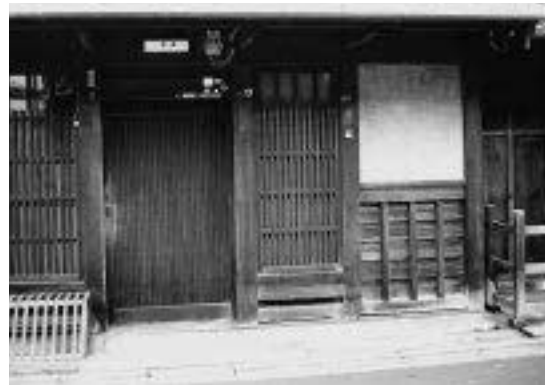
FIG. 65 ARCHITECTURAL ELEMENTS OF THE SUGIMOTO HOUSE: KŌSHI , LATTICE, DOOR; HIRAKŌSHI , FLAT LATTICE WINDOW, TSUCHI , PLASTERED WALL, KŌSHIKABE , 'HIPS' WALL, INUYARAI , DOG'S FENCE. RS.
