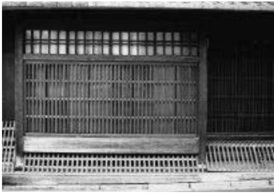
FIG. 64 ARCHITECTURAL ELEMENTS: DEGŌSHI , PROJECTING LATTICE WINDOW AND INUYARAI , A LOW BAMBOO FENCE. THE SUGIMOTO HOUSE. RS.
