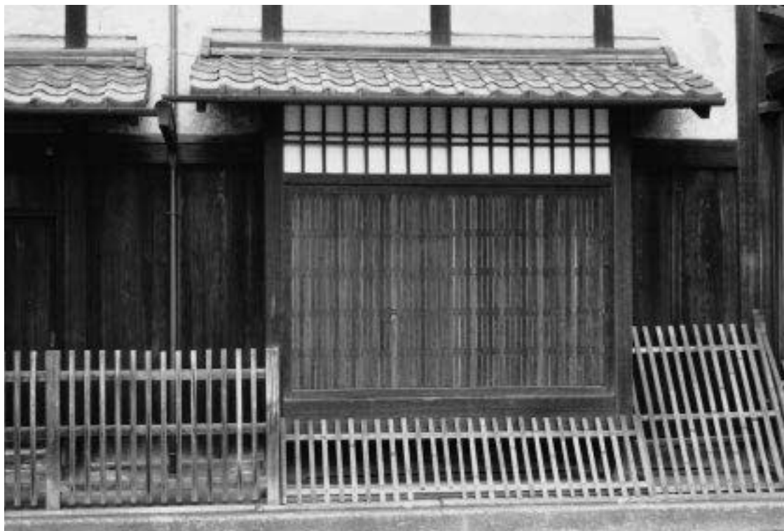
FIG.66 ARCHITECTURAL ELEMENTS OF THE SUGIMOTO HOUSE. DEGŌSHI, PROJECTING LATTICE WINDOW AND INUYARAI, A 'DOG'S' FENCE. RS.
