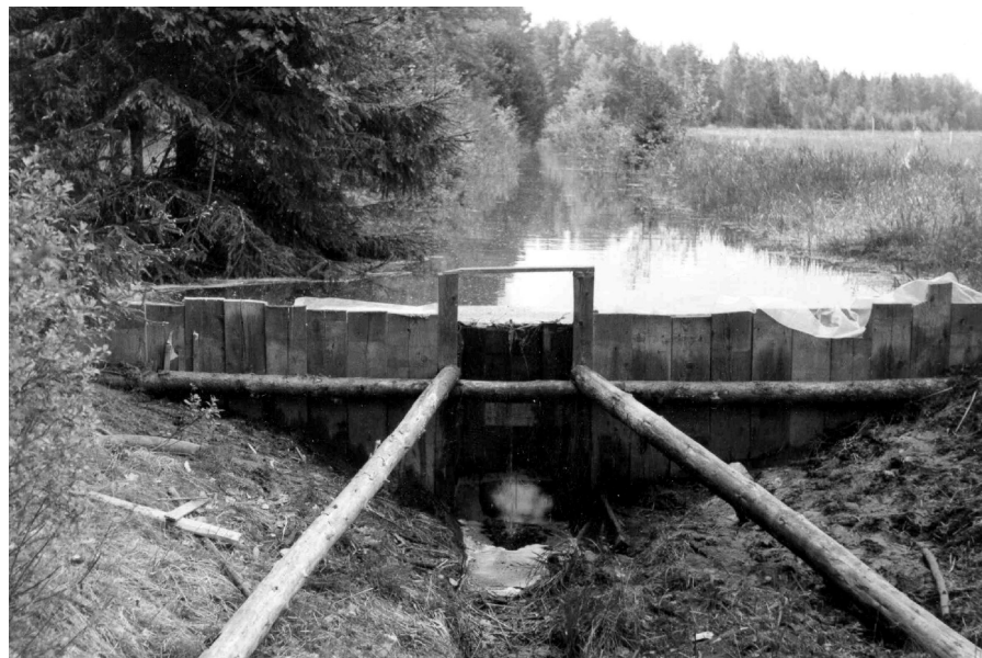
Figure 5.2. Water table regulator on the main ditch.
