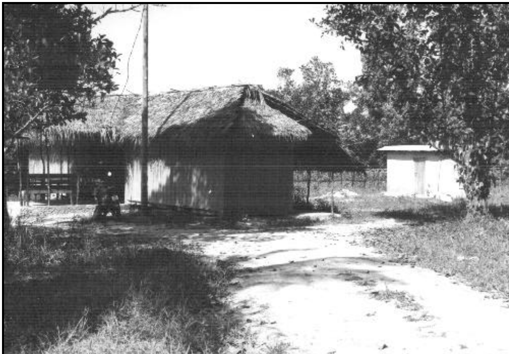
Figure 9.2. A temporary office on the Pemba pilot area
