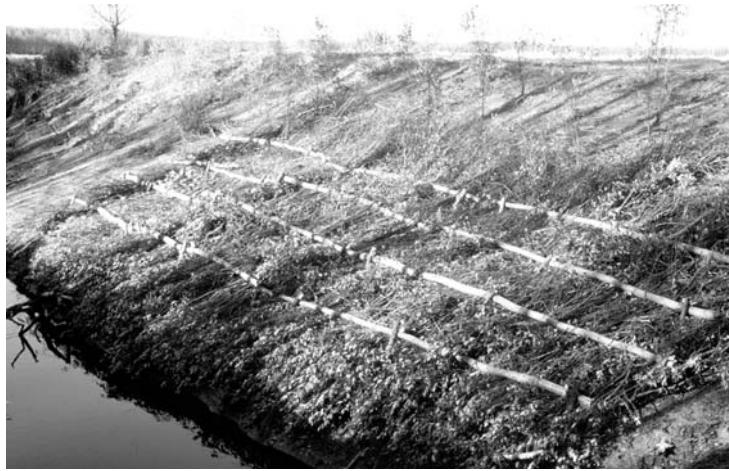
Fig. 3. Example of applying brush mattresses in reach P2 of the Pöntäneenjoki.
