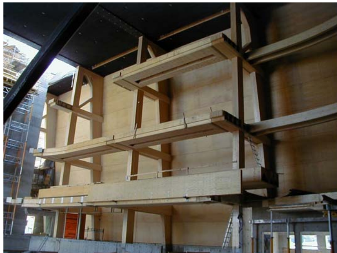
Figure 3. The Sibelius Hall in Lahti, Finland, is a good reference of the integrated use of Kerto-LVL as a sub-product (source: Finnforest).
