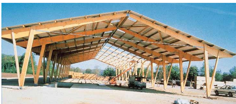
Figure 92. Warehouse in Lengerich Germany with a span of 18 m, made by Barkmann Holzbau GmbH.
