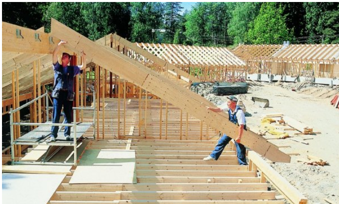
Figure 87. Typical use of Kerto-LVL as a ready-made roof joist component in terraced houses (source Finnforest).
