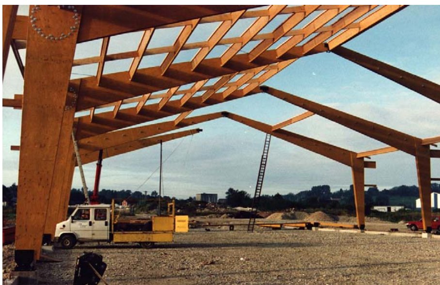
Figure 95. Warehouse in France made by Cordonnier S.A. with Kerto-LVL portal frame and Nordex I-joist (source: Finnforest).
