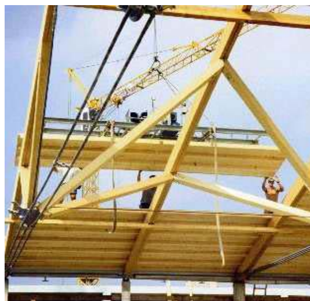
Figure 93. Roof construction of School Nord in Aichach Germany made by Merk Holzbau GmbH. The roof elements are screw glued using Kerto-LVL-Q as a panel and Kerto-LVL-S as ribs with spacing of 600 mm.
