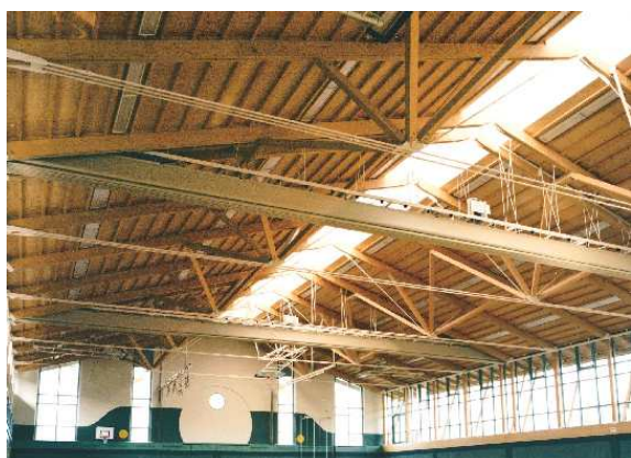
Figure 93. Roof construction of School Nord in Aichach Germany made by Merk Holzbau GmbH. The roof elements are screw glued using Kerto-LVL-Q as a panel and Kerto-LVL-S as ribs with spacing of 600 mm.
