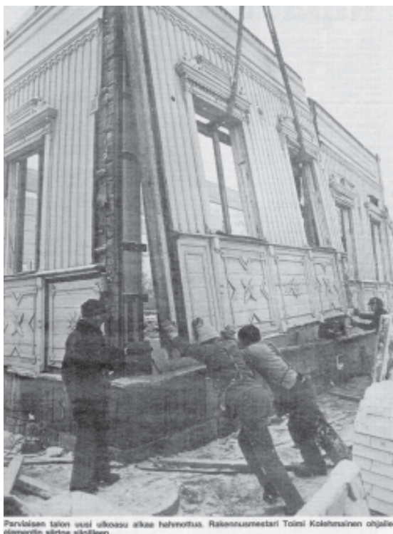
Fig. 23. Taking down the Parviainen house in 1979. The exterior walls were later erected in the 'Ranta-kortteli' area.
