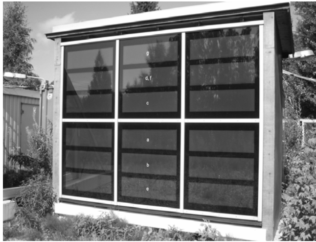
Figure 1. Vertical array of six single-junction a-Si modules in a retrofit BIPV façade installed southwards on the side of a wooden container in Espoo, Finland. Locations of temperature sensors a-g are shown.
