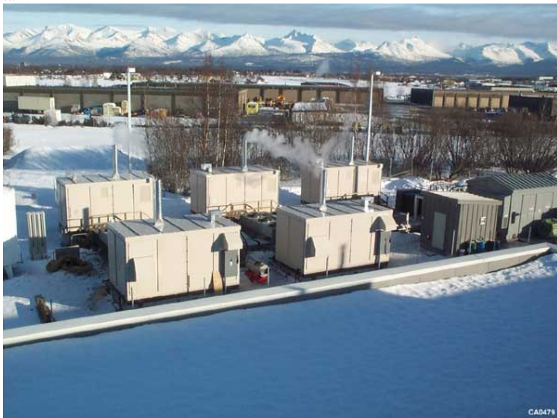
Figure 2.5. a. The PureCell Commercial Fuel Cell Power System - Model 200 from UTC Power (200 kW); b. The PureCell station in Anchorage, USA (Courtesy of UTC Power).
