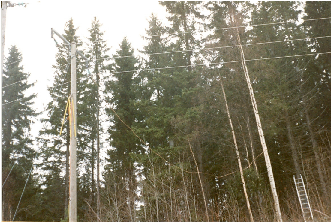
Figure 5.7 The tree as a fault object wired by the network conductor.
