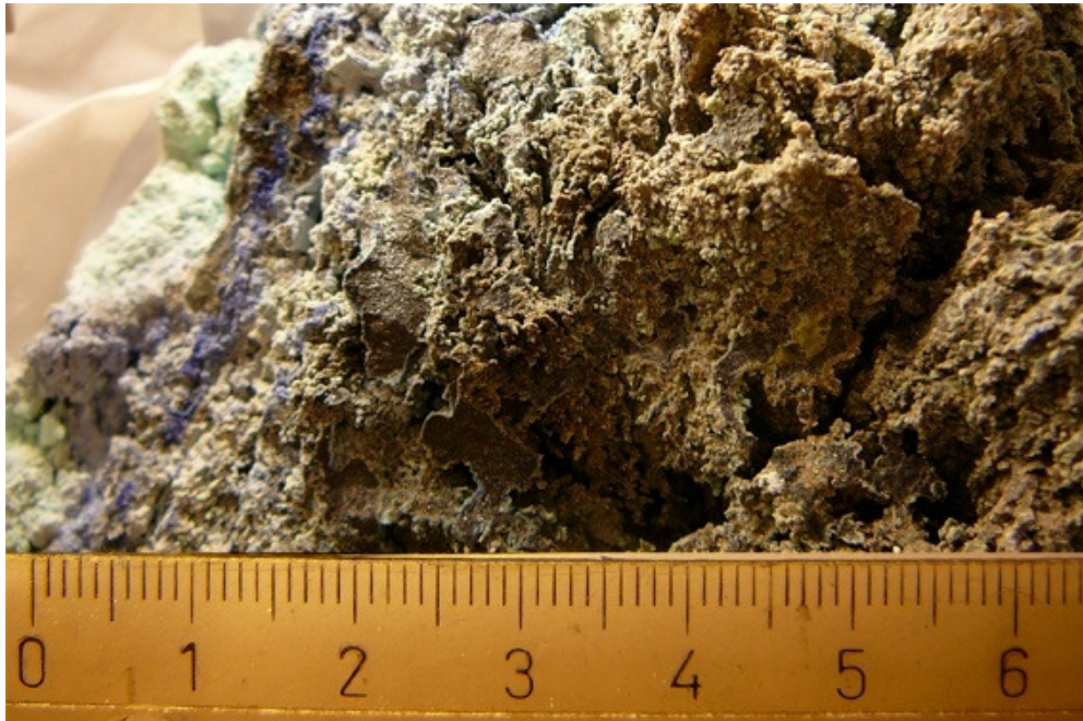
Figure 42. Flue dust build-up sample from the radiation section of the boiler. Sample IV
