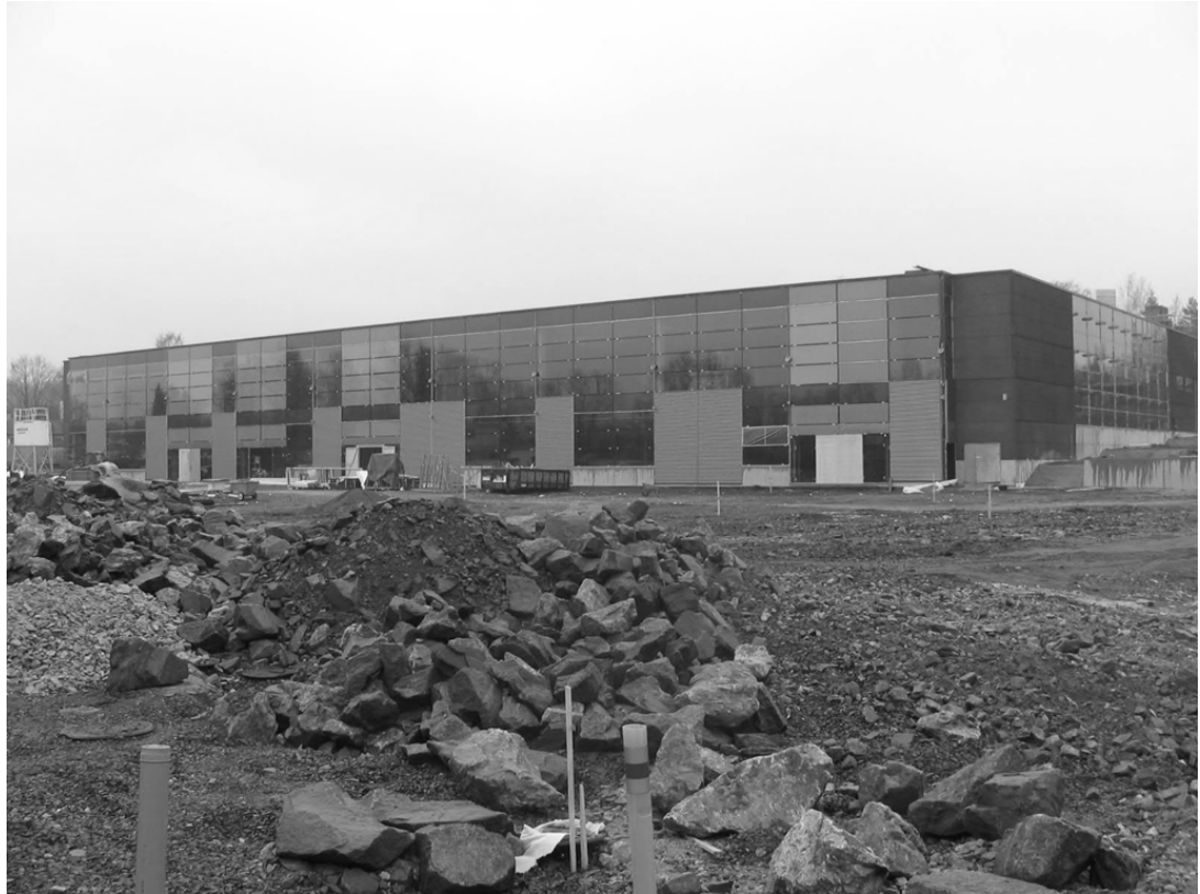
Figure B-1: Glomson retail park was structurally simple box-shape building
