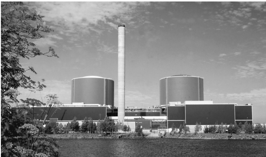
Figure 13: Loviisa nuclear power plant represented the first use of nuclear power technology in Finland. Source: Fortum.
