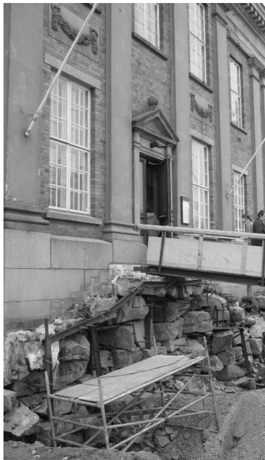
Figure 1 The pilework reparation work of Turku main library
