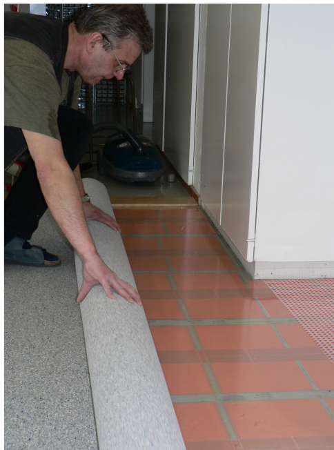
Figure 21. Test room installation on April 28, 2006.
