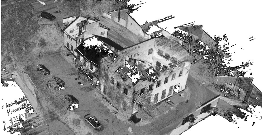
Figure 28. Point cloud data collected with AKHKA for urban renovation.
