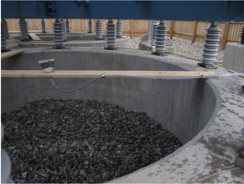
Figure 2.34. Tube extender installed below a reactor
