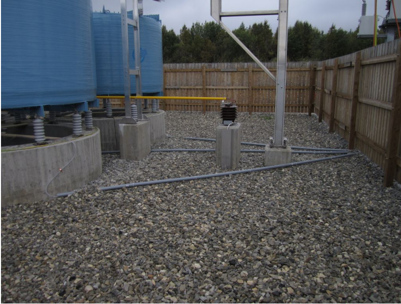
Figure 2.36. Drainpipes protecting the tube extender up to the safety fence
