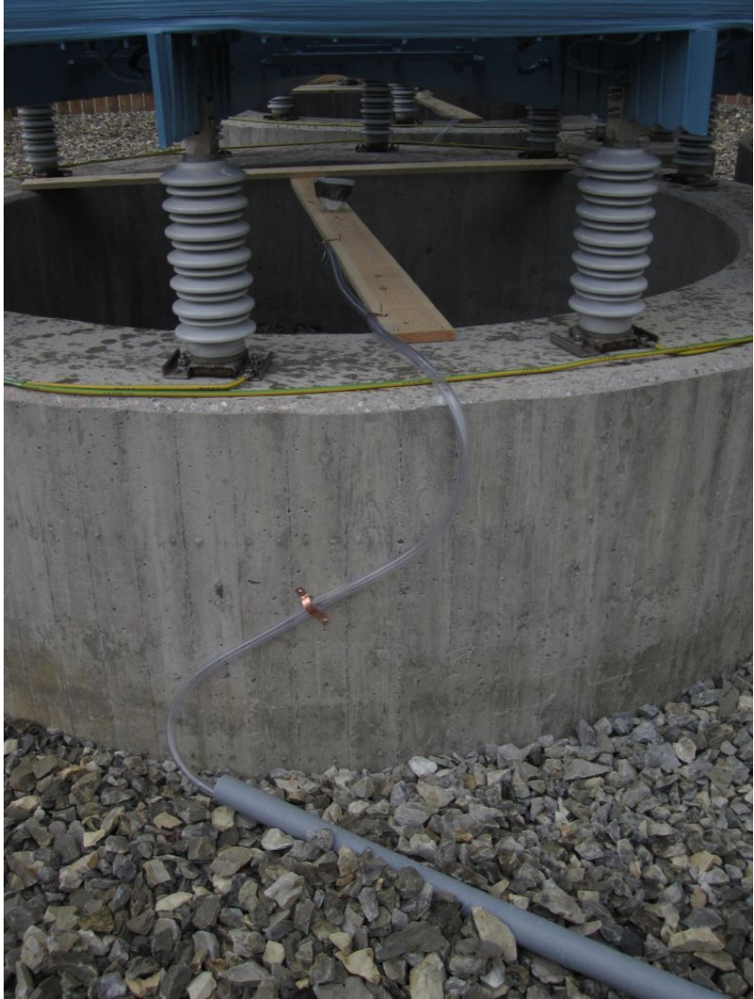
Figure 2.35. Soft tube attached to the concrete below the reactor
