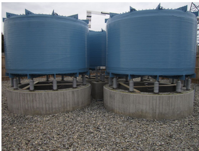
Figure 2.33. Overview of the reactors from the side with the tube extender installed
