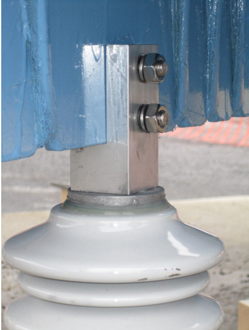
Figure 2.42. Insulator's bolts were loosened to create a minor fault
