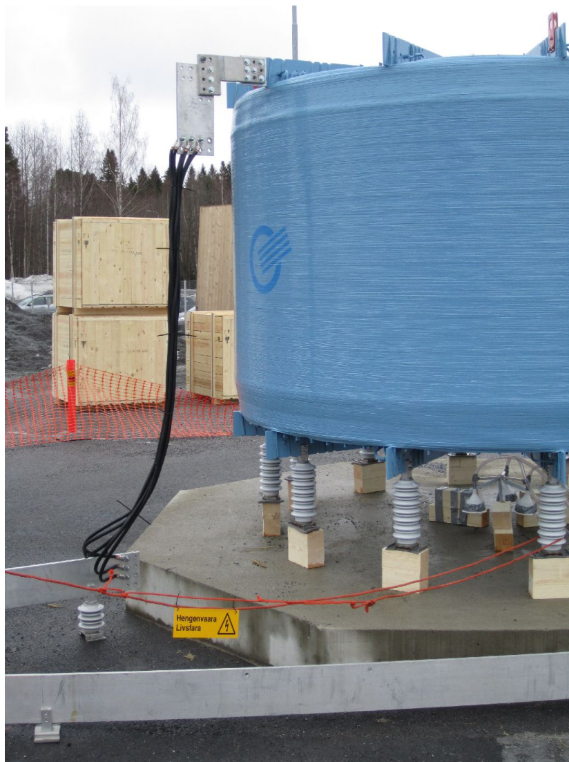
Figure 2.40. Cable ties were used to minimize the vibrations of the input cables
