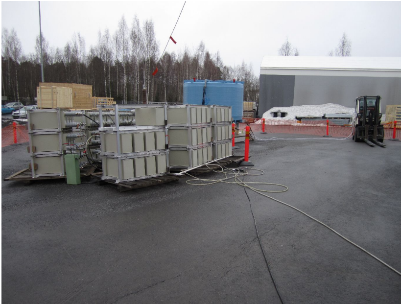
Figure 2.39. Capacitor battery that was used to compensate the reactor being measured
