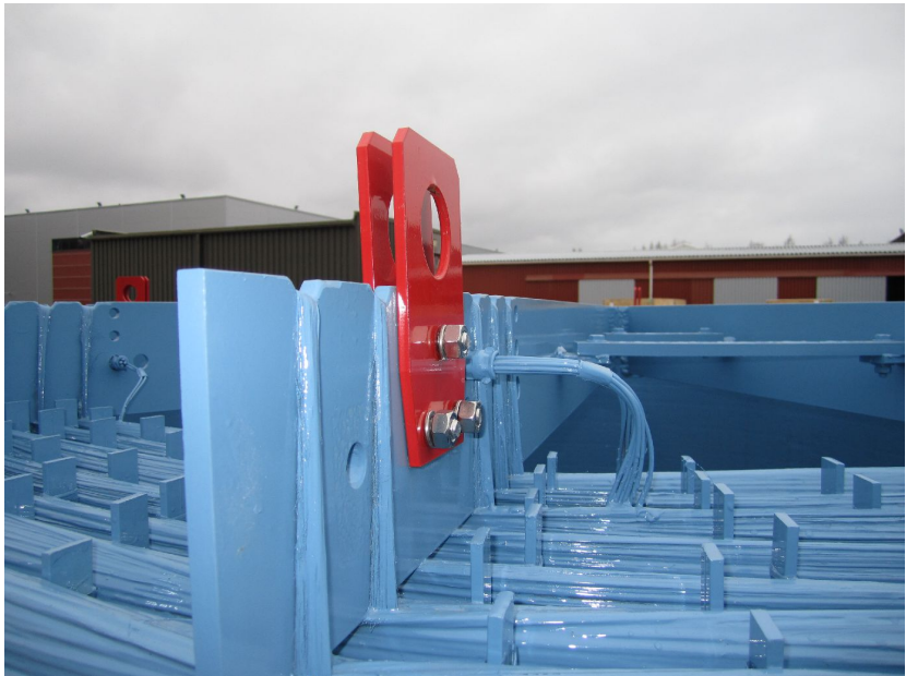
Figure 2.46. Lifting lug's bolts were loosened to create audible noise
