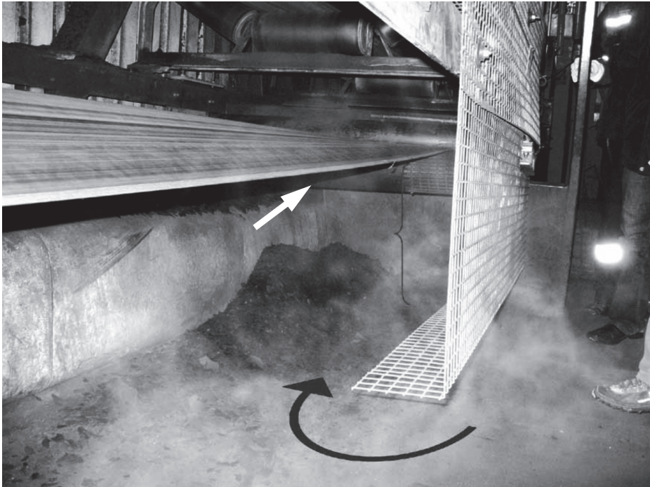
Figure 20. Due to repeated disturbance of belt operation, a fuel supply operator went below the moving conveyor belt to clean the belt turning roller and was fatally caught between the belt and the roller. The location was covered by a steel fence, but it was possible to bypass it during operation. The space between the floor and the lower roll is about 70 cm (TVL/TOT 2009).
