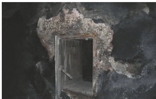
Figure 10. Inside appearance of the bottom maintenance door opening after a smouldering fire in the silo. Photo: Juha Sipilä/Helsingin Energia
