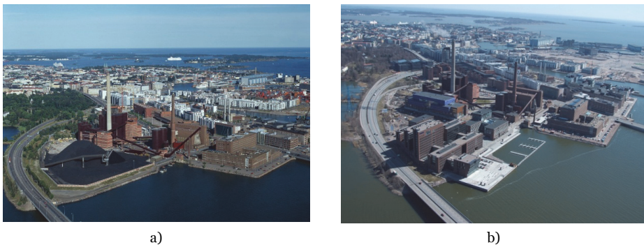
Figure 1. Salmisaari power station a) before and b) after construction of the underground coal storage facility. Photos: Helsingin Energia
