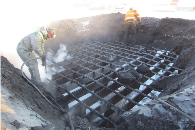
Figure 14. Steam thawing (here almost completed) of a harbour hopper blocked by frozen coal; note residual frozen lumps on the grille. Photo: Juha Sipilä/Helsingin Energia (Publication VI).
