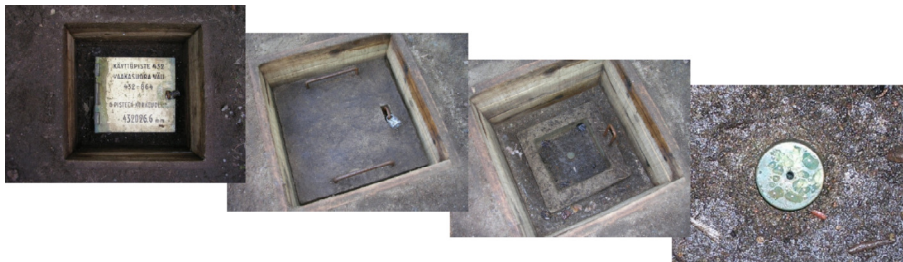
Figure 4.23 The baseline lengths in the final results are the distances between the centres of the holes in the benchmark bolts of the underground markers, reduced to a reference height level.
