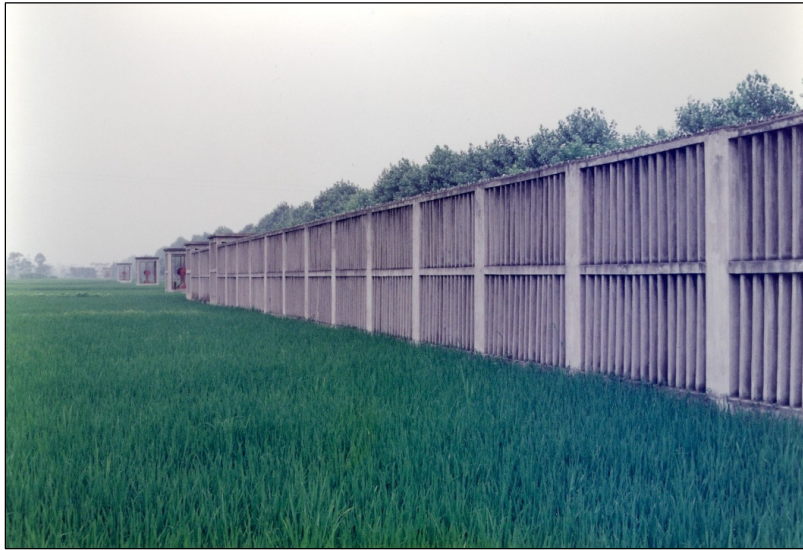
Figure 5.2 The central part of the Chengdu Standard Baseline in November 1998, showing the 50-m-long concrete shelter between pillars 3 and 5.
