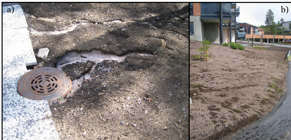
Figure 56. Examples of surface runoff from pervious surfaces at the developing SR catchment: a) surface runoff from pervious surface near manhole in July 2004, b) soil and newly sowed grass seeds were washed off from a compacted pervious slope during a rainfall event after landscape works in May 2006.
