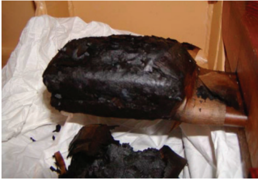
Figure 5-14 Power transformer incipient fault detected with off-line diagnostics in 2003.
