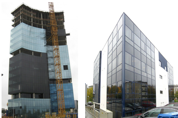
(a) Cast SFRC floor-slabs in Rocca Tower, Tallinn, Estonia. (b) Cast SFRC floor-slabs in the office building on Kotkapoja street, Tallinn, Estonia.
