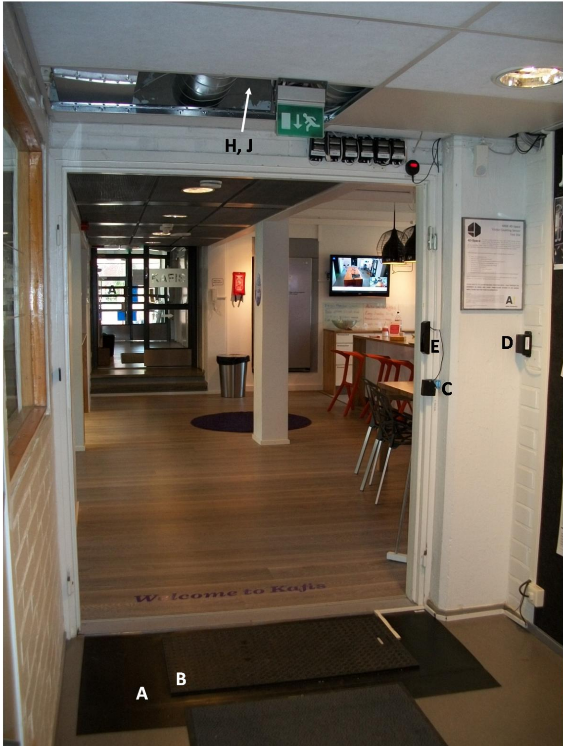
Figure 39. Test site as seen from the corridor. Sensors: A Emfit, B Schmersal, C Clas Ohlson, D Takex, E Cedes, H Eurotech, and J Axis.
