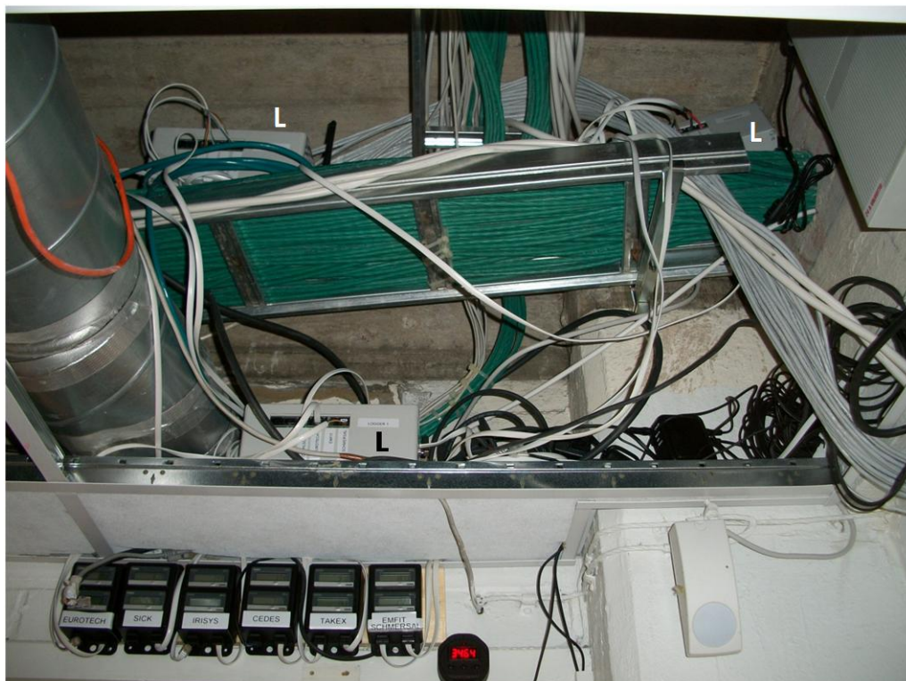
Figure 51. Visit Log 4000 GSM data loggers (L) and hardware cabling placed above the detachable ceiling panel on the corridor side. One logger is missing from the picture.
